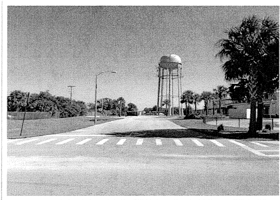
View of North Entrance to School District of Indian River County's Property and Subject Parcel's Potential Ingress/Egress Easement from 28 th Court – Facing East
